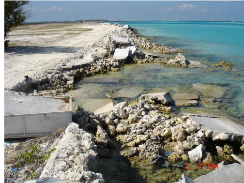
(b) Completely collapsed Seawall
