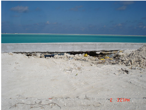
(a) Void caused by through-wash of drainage
