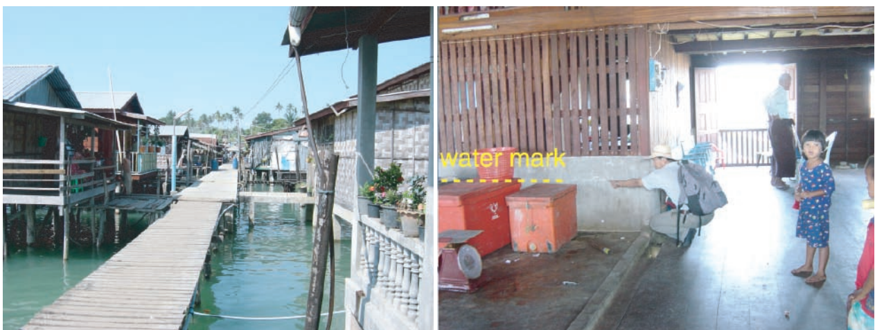
Photo 10. Houses above water (left) and the watermark on the wall of a house (right).
