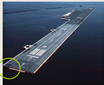
Mega-Float Phase-II model (1000m × 60~120m × 3m/1m)
