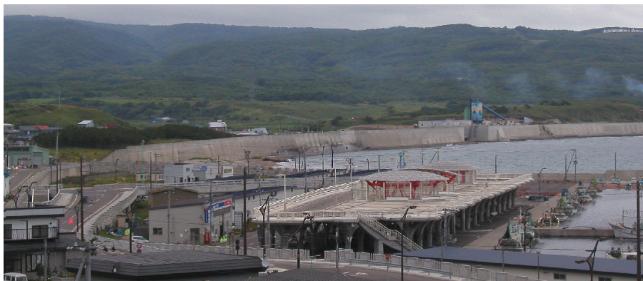
Photo 5.1.2 Tsunami evacuation terrace
